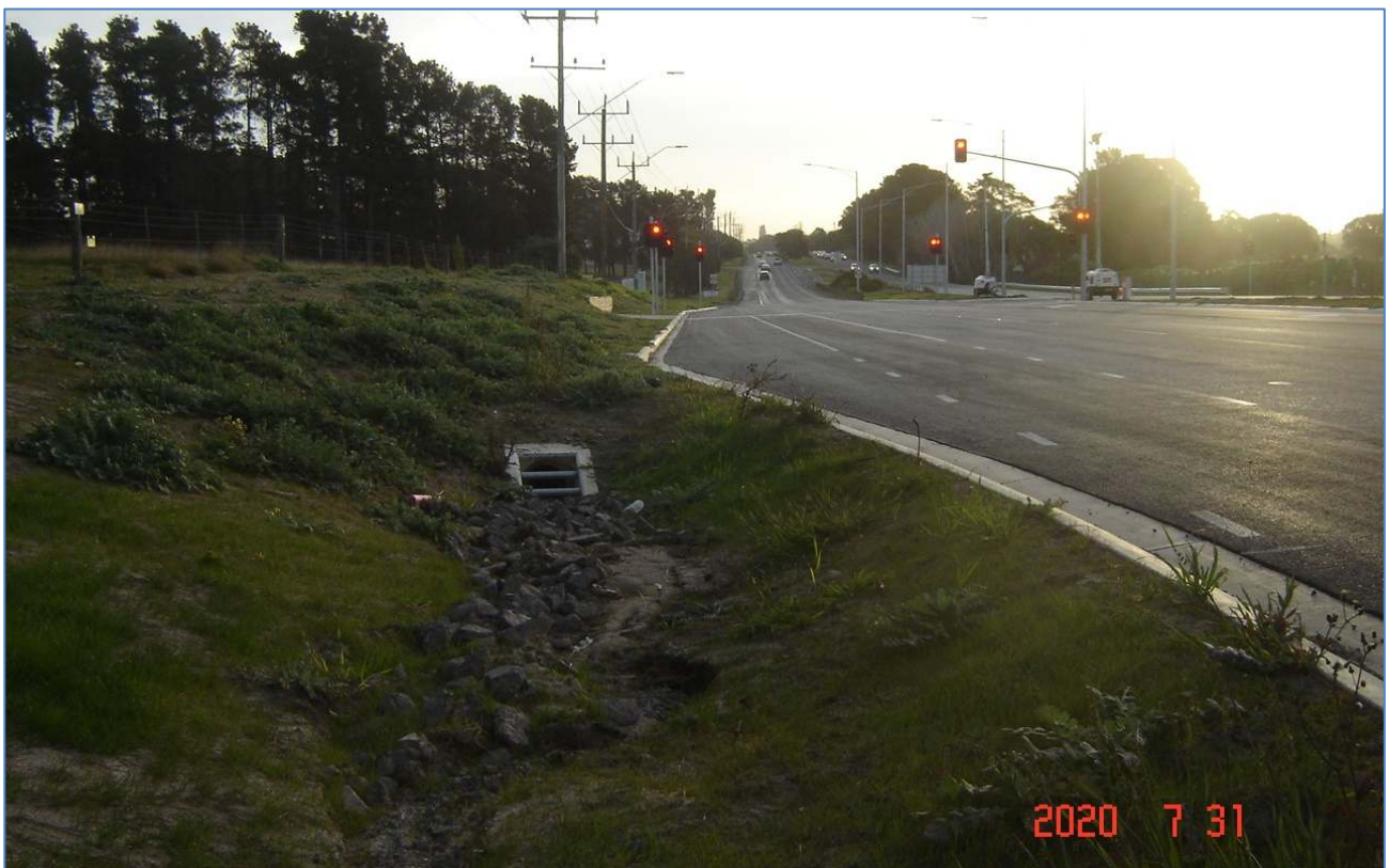
Culvert on east approach with steep batter from back of kerb?
