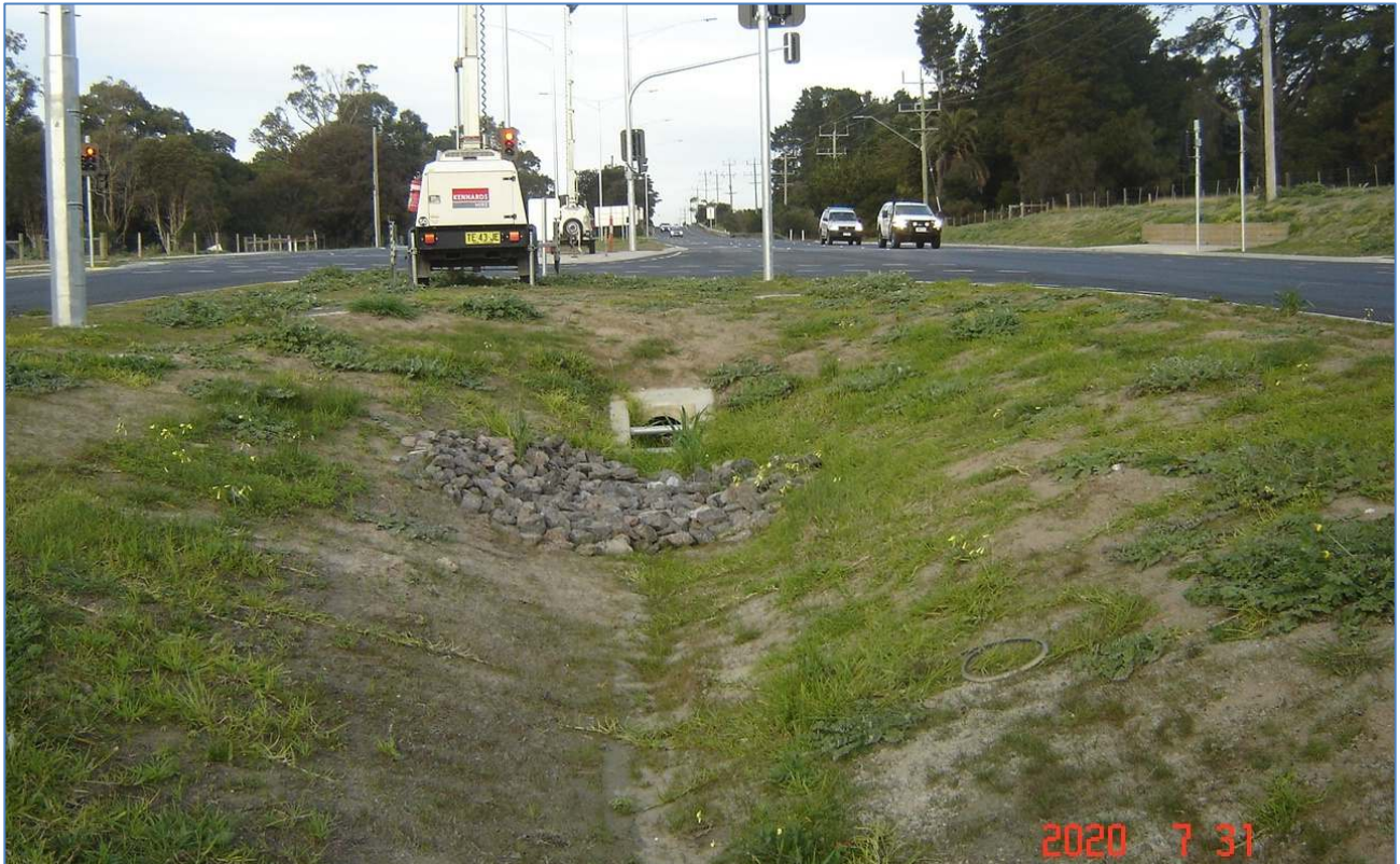
Steep batters to culvert endwall -worst case is south side for west bound traffic.
