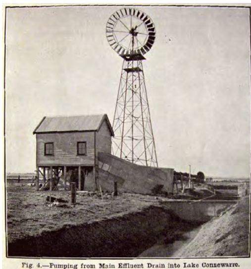
Photo 4: The big windmill and the weatherboard building housing the centrifugal pump. ("Sparrovale Farm, Marshall", Ferguson, Investigator - Magazine of the Geelong Historical Society, Vol 28, No 3, September 1993)
