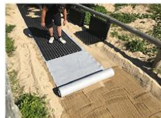
Gravel with erosion control matting
