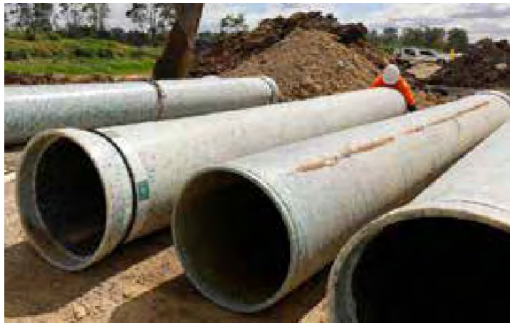
Figure 1.73 Recycled plastic drainage pipes used in Victoria's Big Build. Source: www.bigbuild.vic.gov.au
