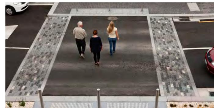
Example of a raised pedestrian crossing with 'rumble' pavement edges and kerb outstands. Taradale, New Zealand
